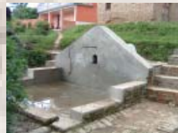
Renovation of public taps for better service
