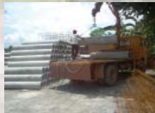
This capital intensive part was supported by UNHABITAT
