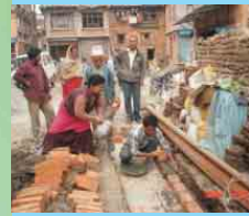
Community people involving in drain construction
