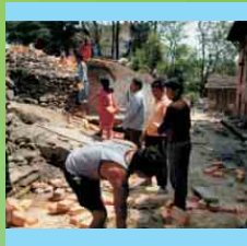
Community people involving in brick paving works
